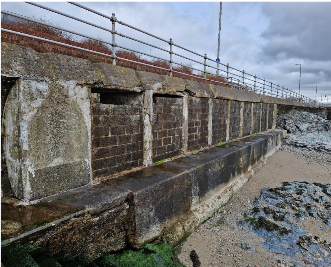
Figure B.10: Walkway in front of Victorian changing rooms
