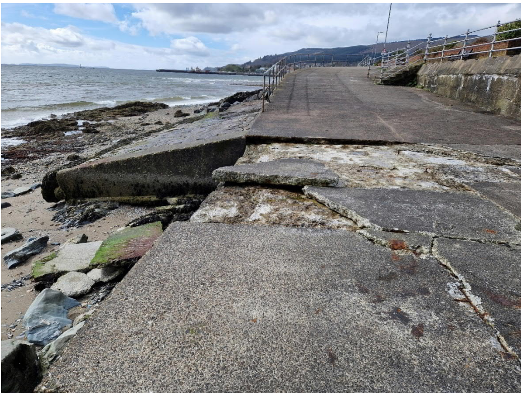
Figure B 2: Paved revetment and access ramp
