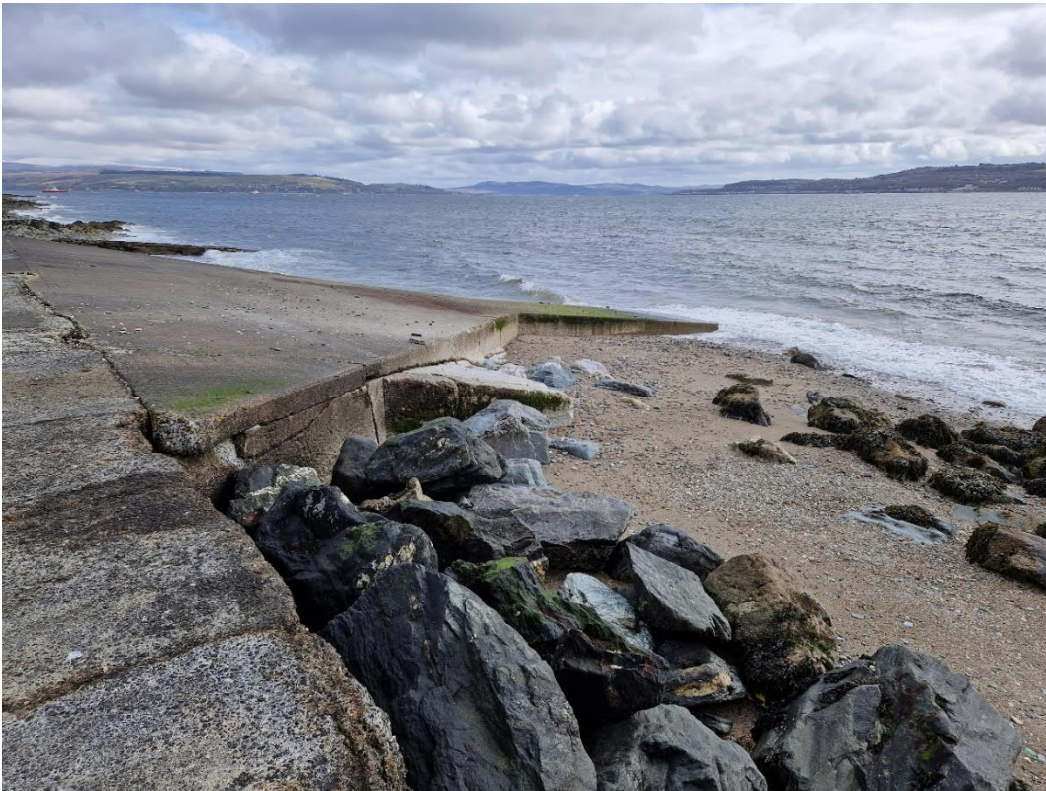
Figure B.7: Concrete slipway from parking area
