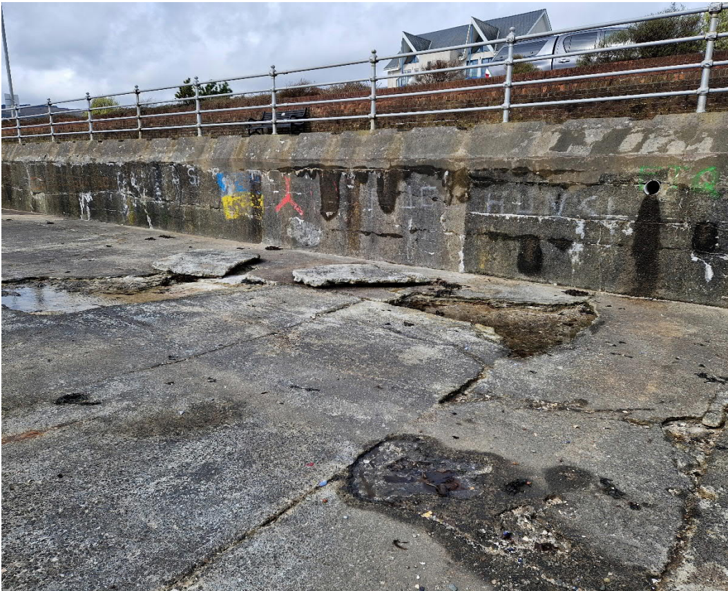
Figure B.5: Wall to the rear of the parking area
