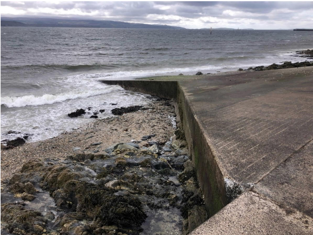
Figure B.8: View of slipway from in front of bathing area
